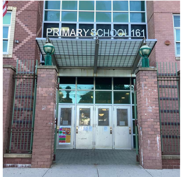
Facade A - 124th Street
