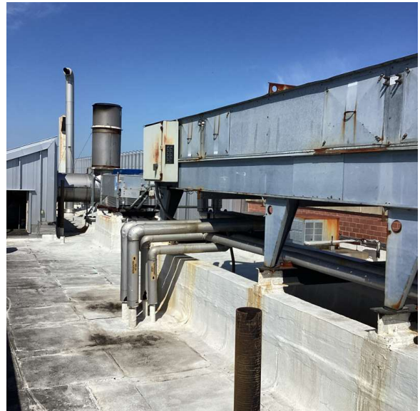
Roof 1 - East view
