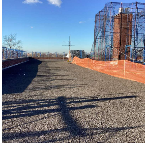
Roof 1 - Southwest View
