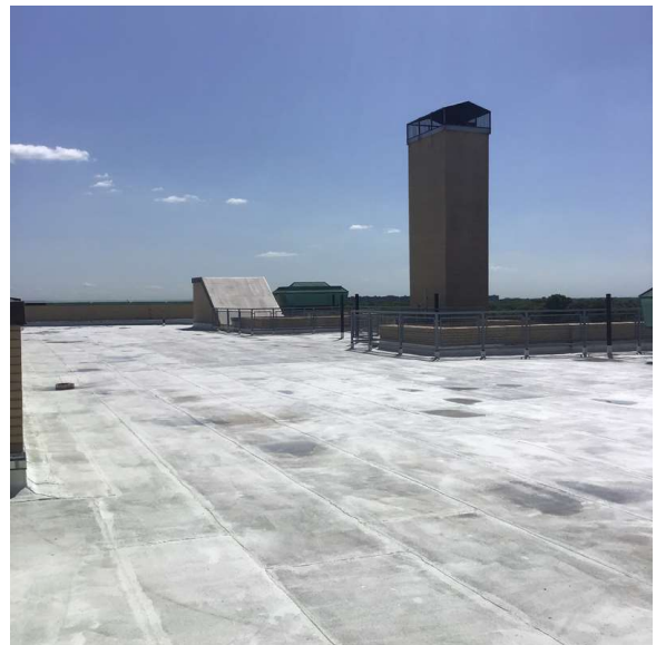
Roof 1 - Southeast view
