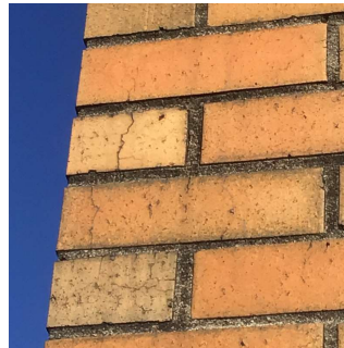
BH2 No violations recorded.
