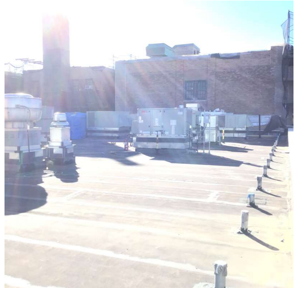
Roof 7 - Southeast View
