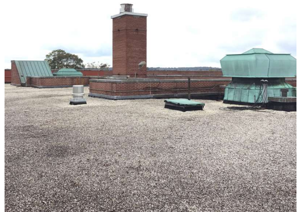
Roof 1 - Northwest view
