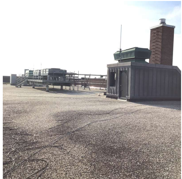
Roof 1 - Southwest view
