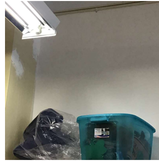
Facade H - Room 115
