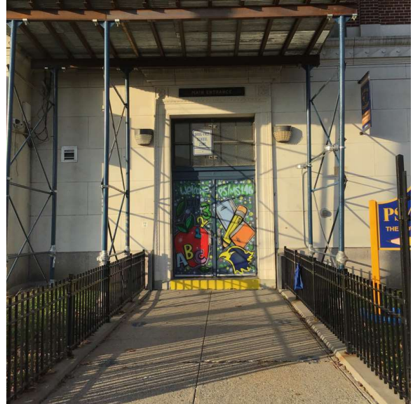
Facade A - 99th Street
