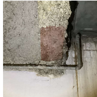
Basement - Ash Hoist Vault
