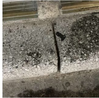
Facade A No violations recorded.
