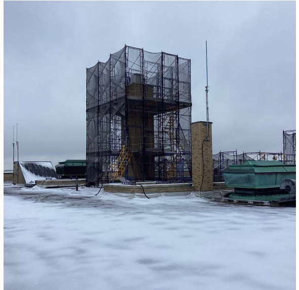
Roof 1 - Southeast view
