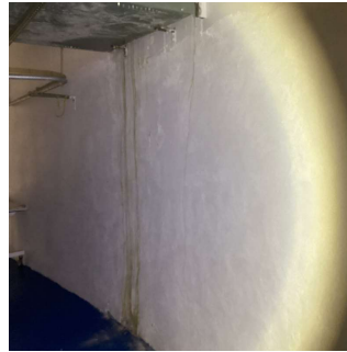
Basement - Electrical Panel Room
