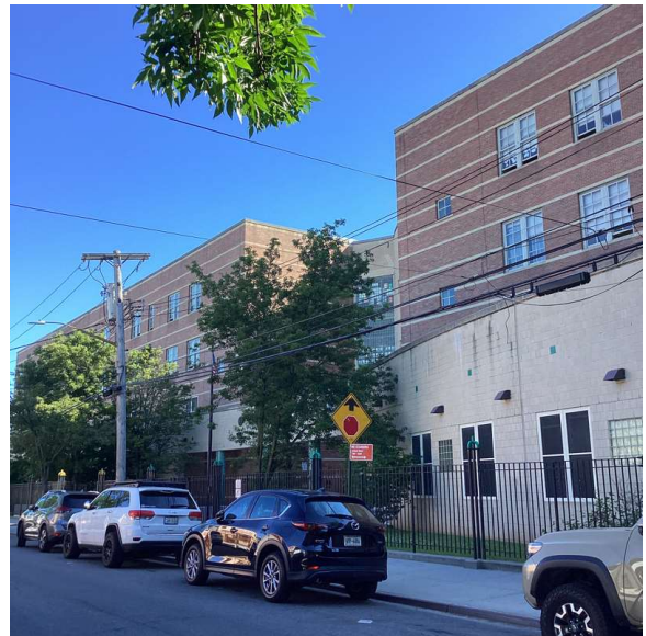
98th Street - Northeast view
