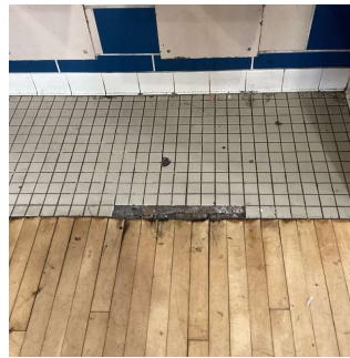
Drinking Fountain Area
