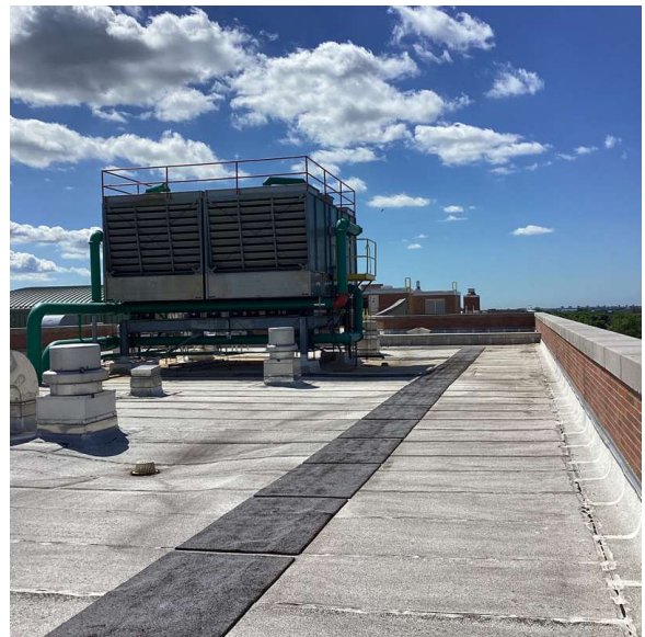
Roof 1 - South view
