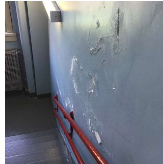
Facade F - Stair C
