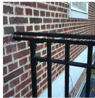
Facade A No violations recorded.
