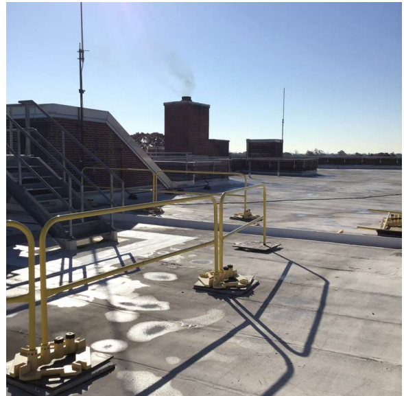
Roof 1 - Northeast view
