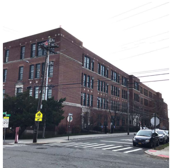
Corner of 7th Avenue and 128th Street - Southeast View
