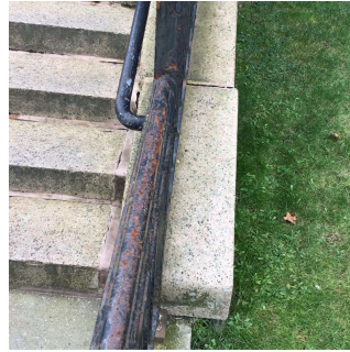
Facade C - Exit 7
