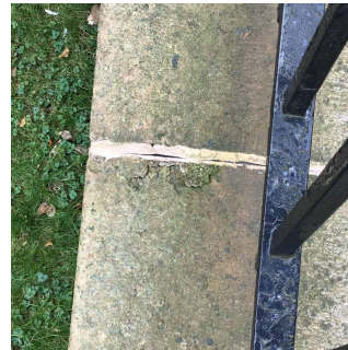
Facade B - Exit 3
