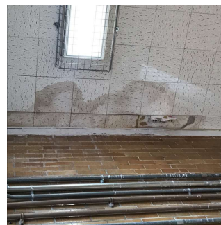
Roof 2 - Gymnasium (Roof 2 - Rooms 352A, 352E similar)
