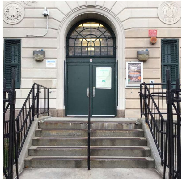
Facade A - 128th Street
