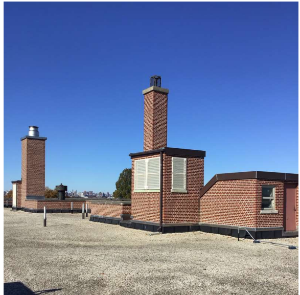
Roof 1 - East View
