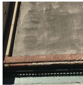
Facade H No violations recorded.
