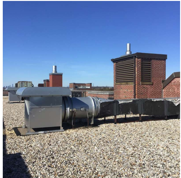
Roof 1 - Northwest view
