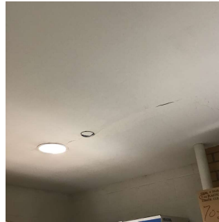
Storage room 104A
