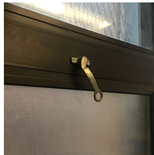
Facade J - Room 161
