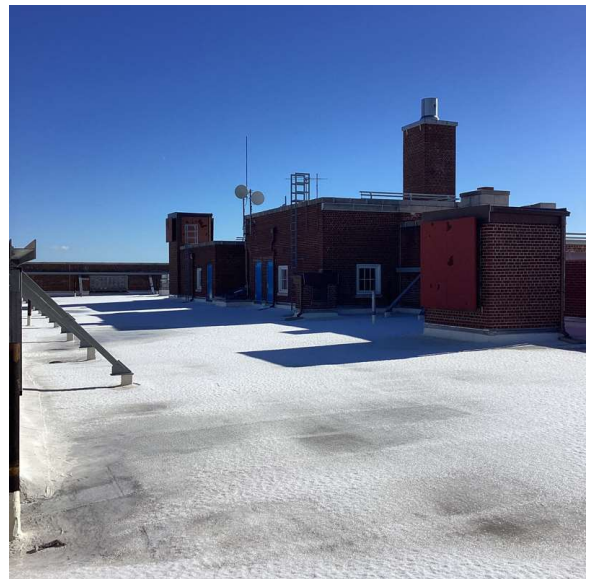
Roof 1 - Southeast view
