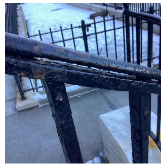
Facade A No violations recorded.
