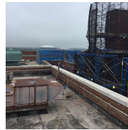
Roof 1 - Northwest View
