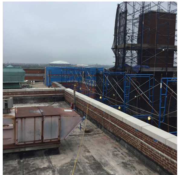
Roof 1 - Northwest View
