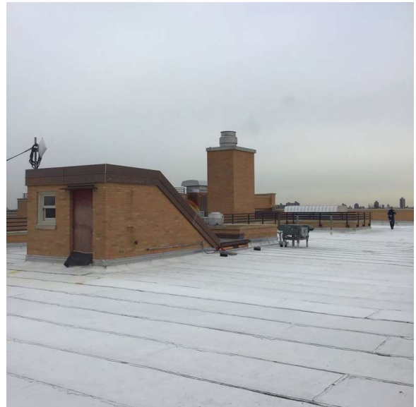
Roof 1 - Southwest View
