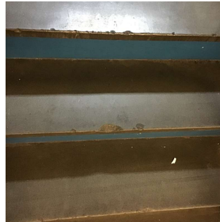
Corridor near Room 119B
