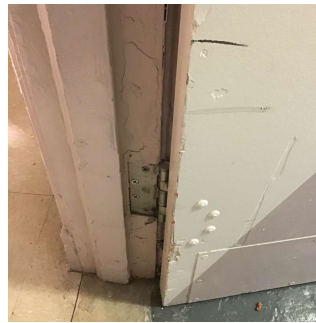
Stair to Dressing Room
