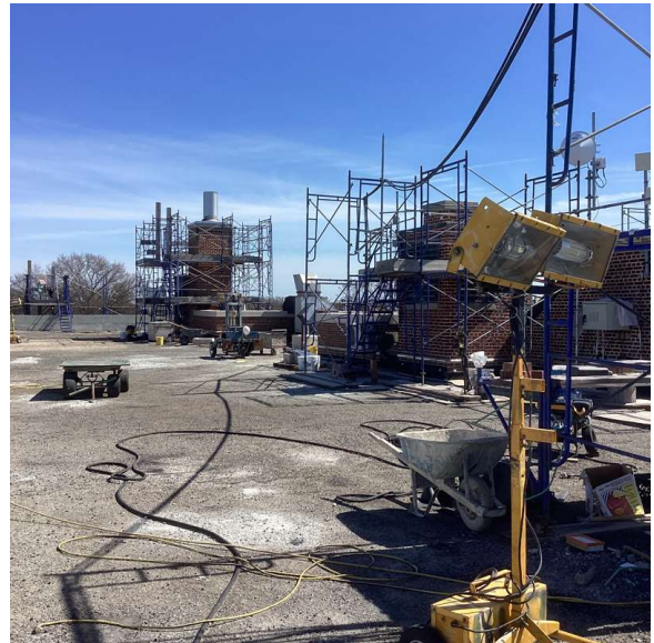
Roof 1 - East view
