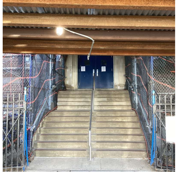
Facade A - 109th Road
