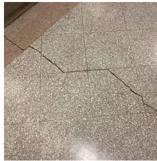
Corridor near Room 161
