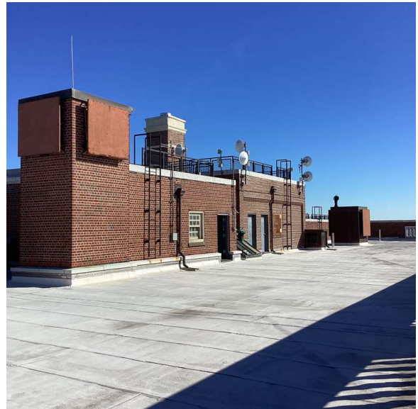
Roof 1 - East view
