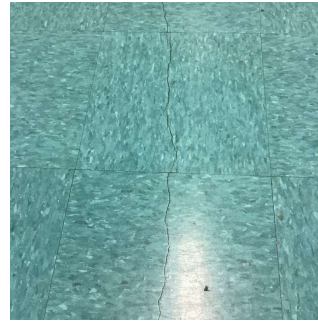
Corridor near Stair C/1
