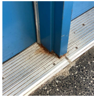
Facade G - Exit 9
