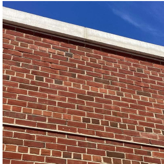
Roof 2 - Facade G
