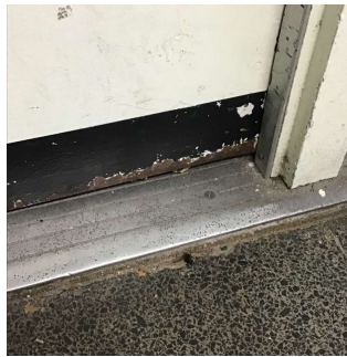
Facade E - Exit 8 No violations recorded.
