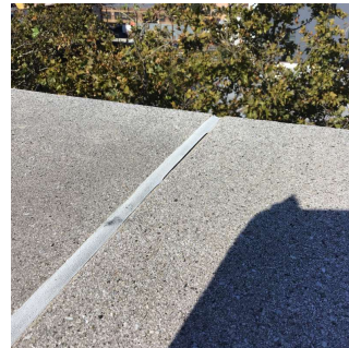
Roof 1 - Facade A
