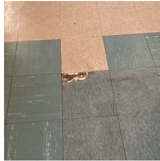
Near Toilet Room
