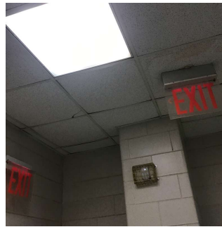
Near Stair E/5
