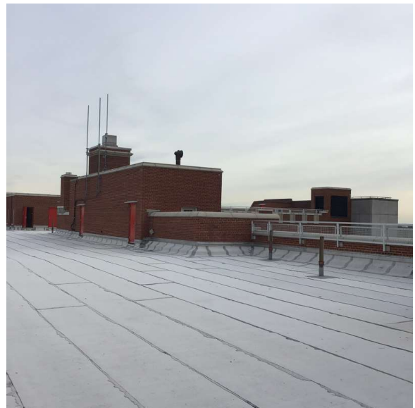
Roof 1 - East view
