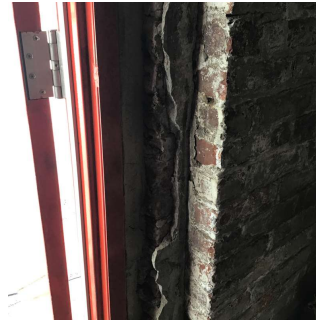
Roof 1 - Tank Room
