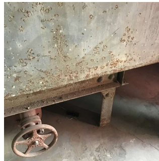
Roof 1 - Tank Room
