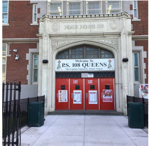
Facade A - 109th Street
