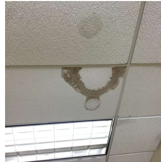
Roof 6 - Corridor near Room 403 (shown), Corridor near Room 408 (similar)
