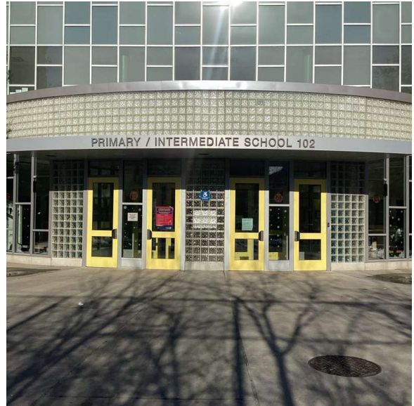
Facade A - Van Horn Street
