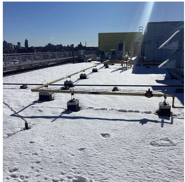
Roof 6 - Southeast View
