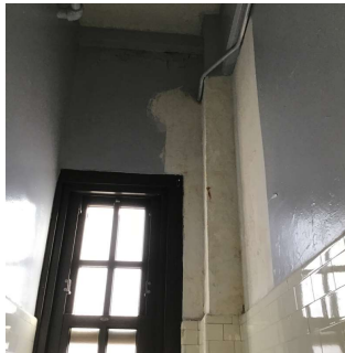
Facade F - 1st Floor Women Toilet Room
