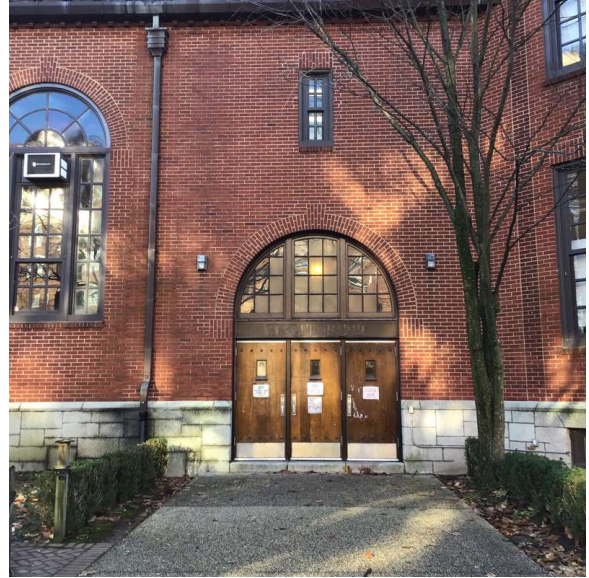
Facade C - Slocum Crescent
