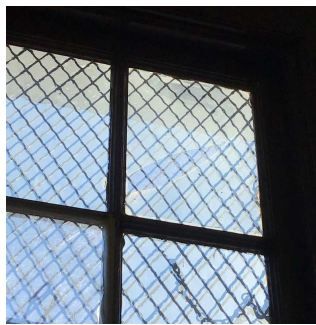
Facade F No violations recorded.
