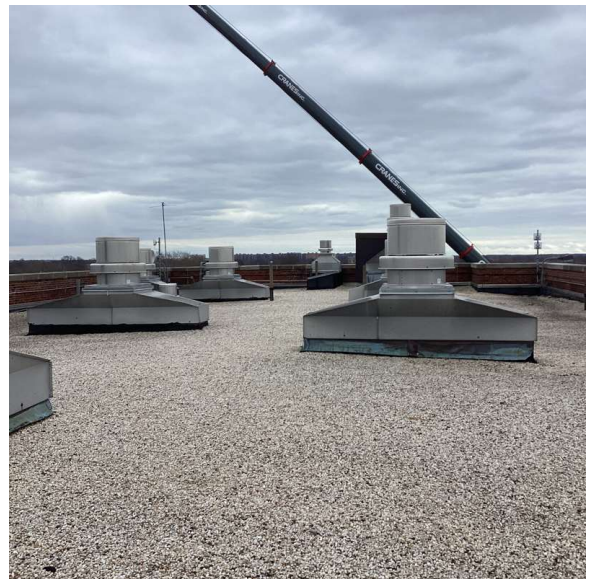
Roof 1 - East view
