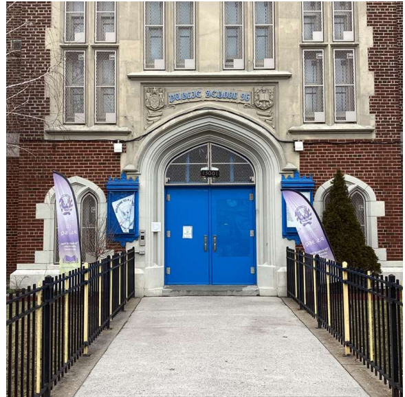
Facade A - Rockaway Boulevard
