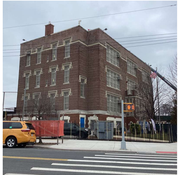
Corner of 130th Street and Rockaway Boulevard - Northeast view
