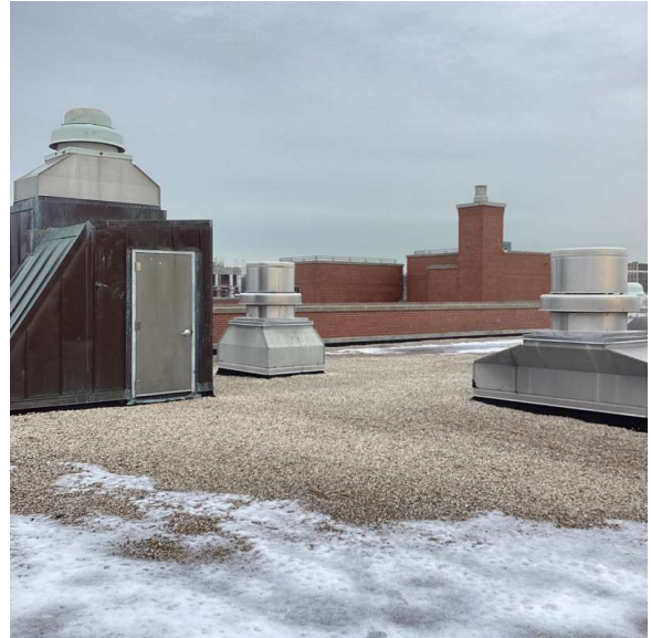
Roof 1 - North view
