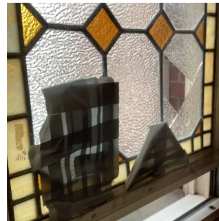
Facade F - Auditorium
