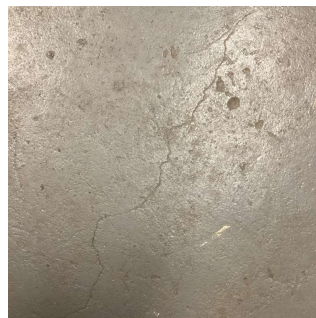
Ground Floor - Water Main
