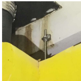
Roof 12 - Gas Meter Room, Sub-Basement Corridor, Boiler Room No violations recorded.
