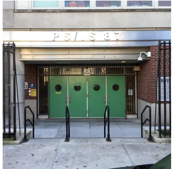
Facade A - 67th Drive
