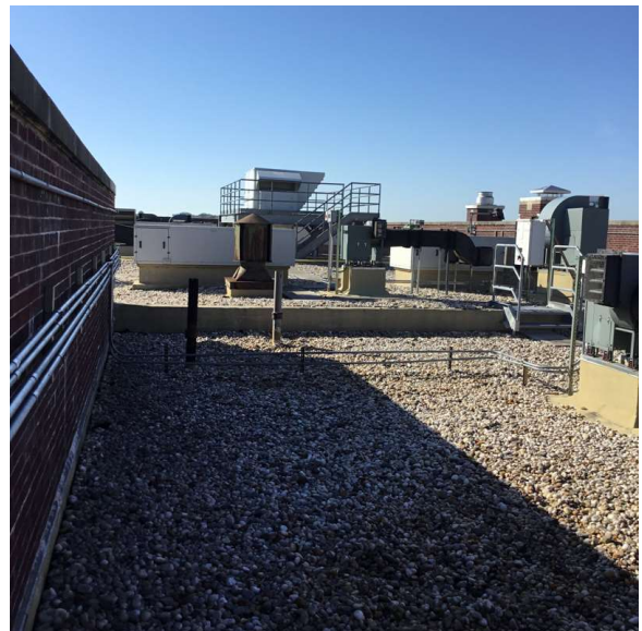
Roof 1 - Southwest View
