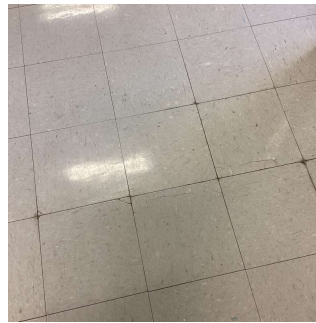
Corridor near Room 104
