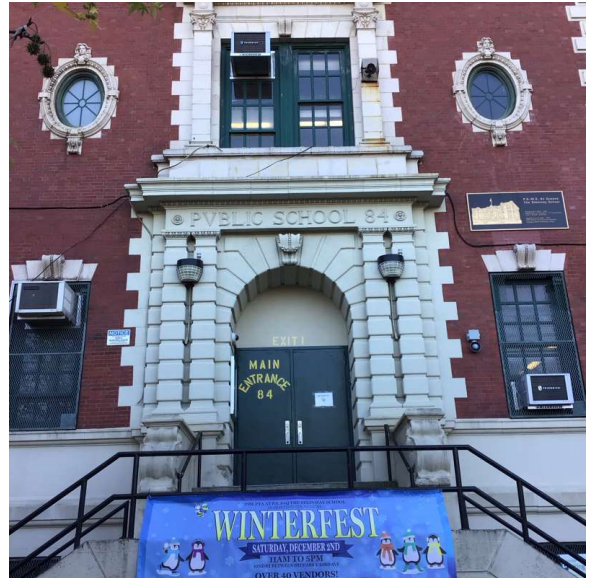
Facade A - 41st Street
