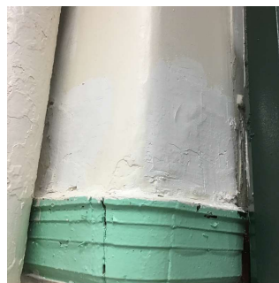
Near Stair D
