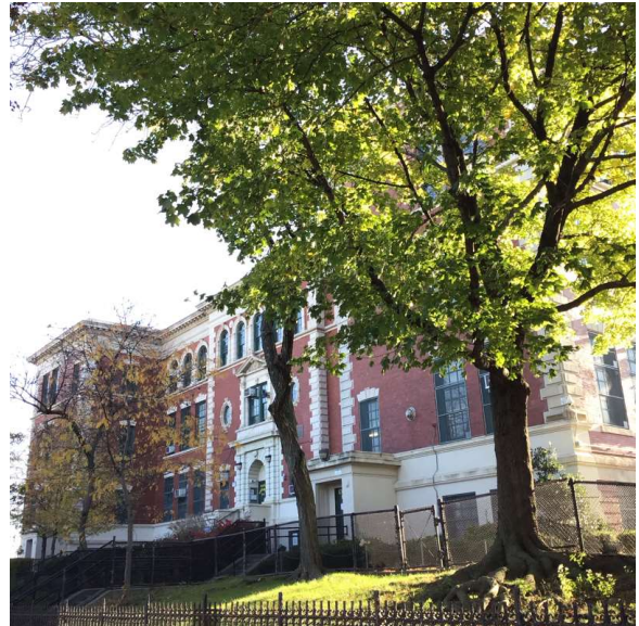
41st Street - West View
