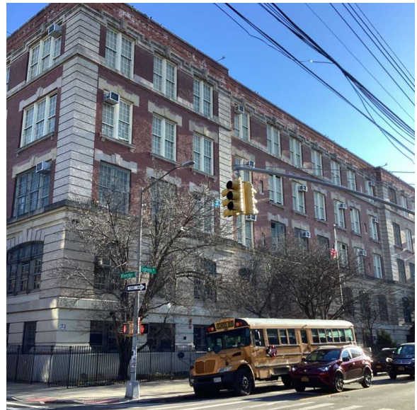
Corner of Bleecker Street and Cypress Avenue - East view
