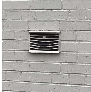
Facade B No violations recorded.
