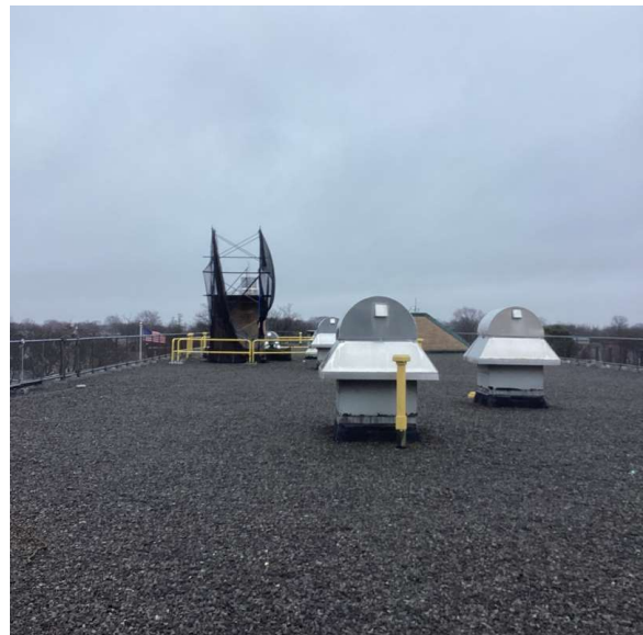
Roof 1 - South view
