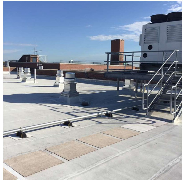
Roof 2 - Northeast View
