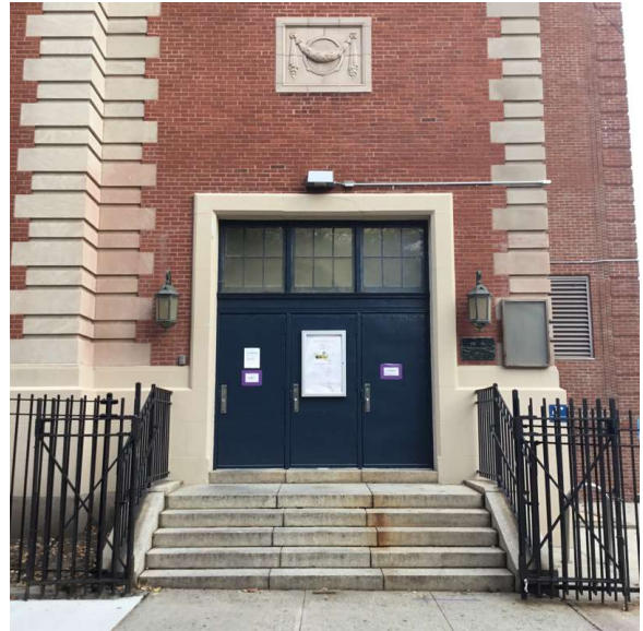
Facade A - 15th Drive
