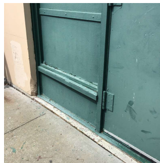
Facade D No violations recorded.
