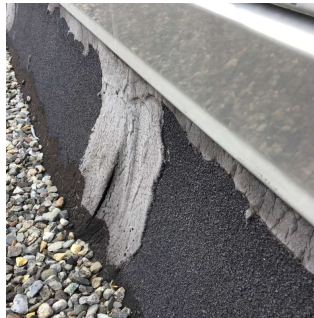
Roof 1 Facade D
