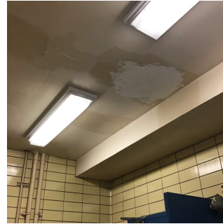
Roof 1 - Stair F/3 No violations recorded.
