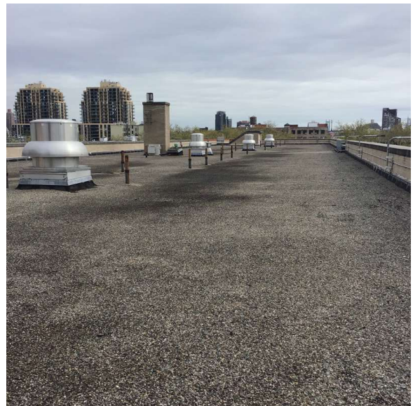
Roof 1 - Northeast view
