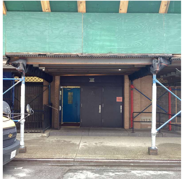
Facade A - Hancock Street
