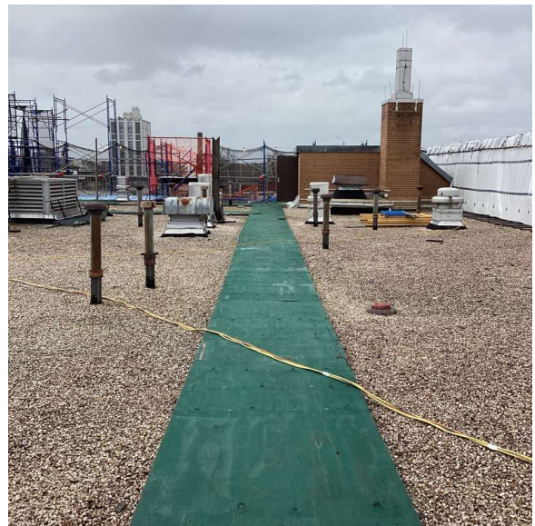
Roof 1 - Southwest View
