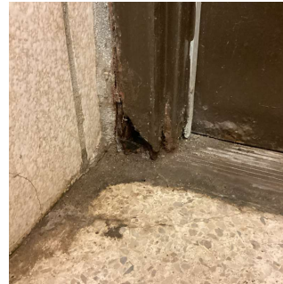
Facade D - Exit 6
