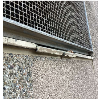
Facade F - Window Sills
