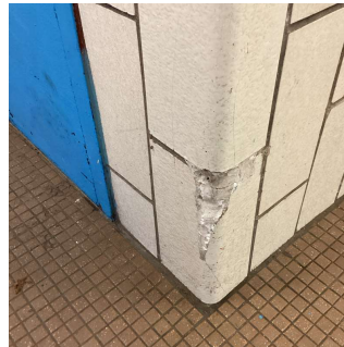
Near Emergency Exit
