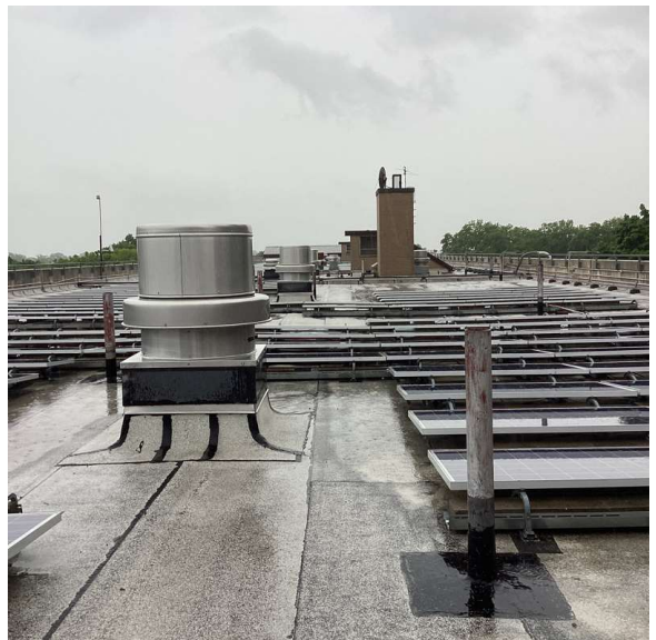
Roof 1 - South view
