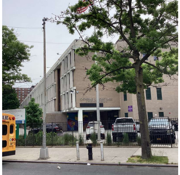
Facade A - Northeast view
