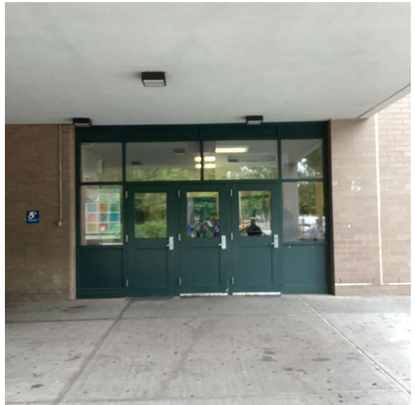
Facade A - Guy R. Brewer Boulevard
