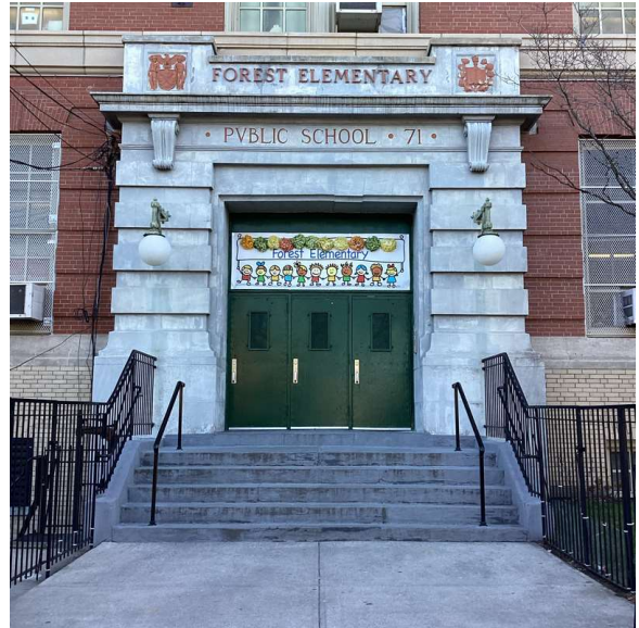
Facade A - Forest Avenue
