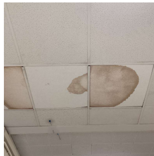
Corridor near Room 327
