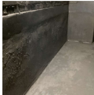
Sub-Basement - Oil Tank Room
