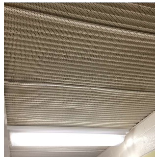
Corridor near Room B19
