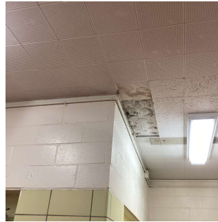
Corridor near Room 116
