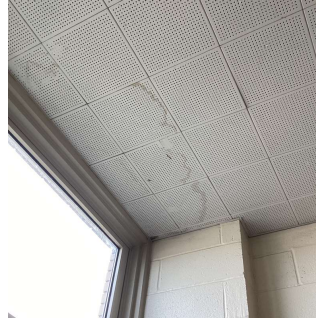
Corridor near Room 216
