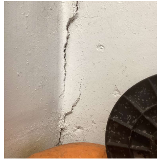
Sub-Basement - Boiler Room
