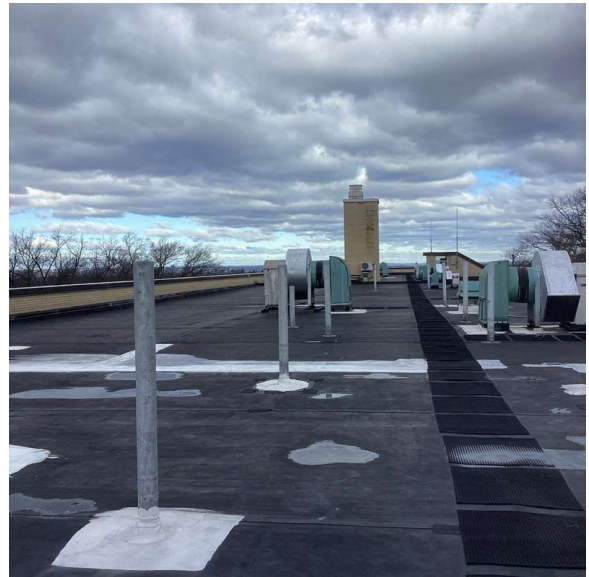
Roof 1 - Northwest view
