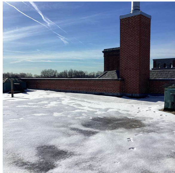
Roof 1 - Southwest view
