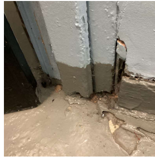
Stair C/Basement Vestibule
