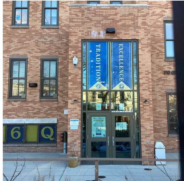
Facade A - 102nd Street
