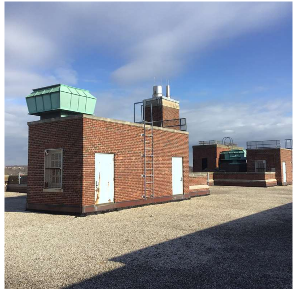
Roof 1 - Northeast view
