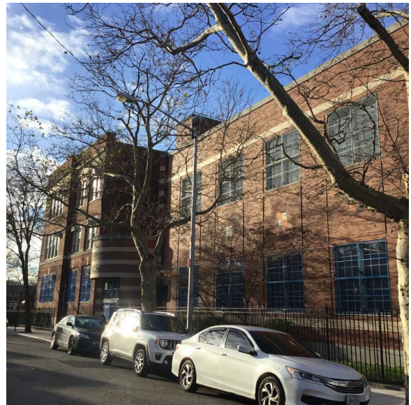
101st Avenue - South view
