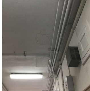
Corridor near room 303A
