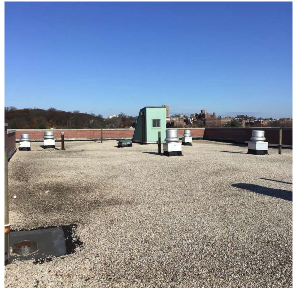
Roof 1 - North view
