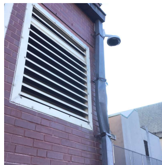
Facade D No violations recorded.
