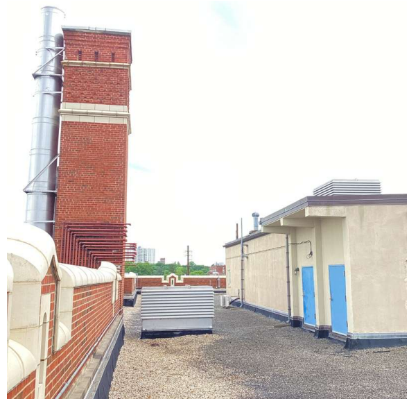
Roof 1 - North View
