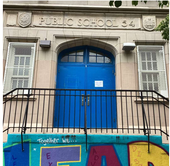
Facade A - 127th Street
