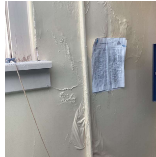
Facade H - Room 401B, also Rooms 401D, 401F, Facade A - Room 113
