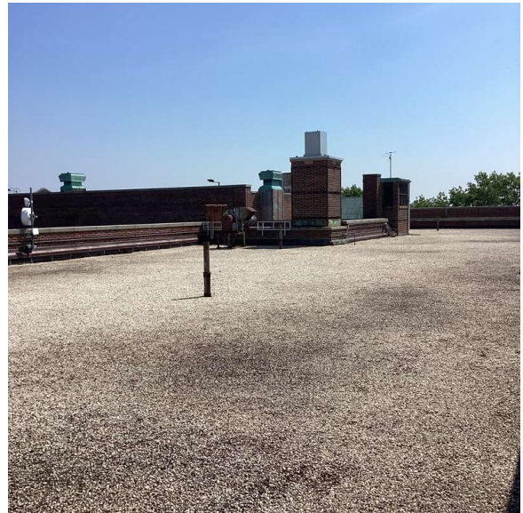
Roof 1 - Northeast view
