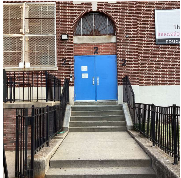
Facade A - 146th Terrace
