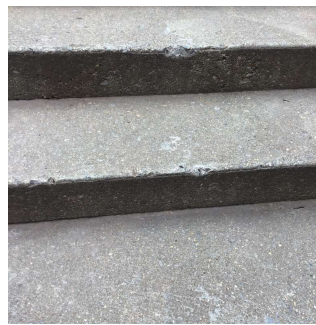
Facade A No violations recorded.
