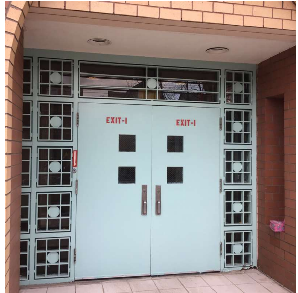
Facade A - 117th Street
