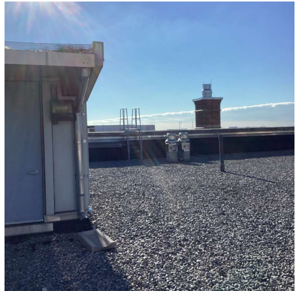
Roof 1 - South view
