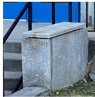
Facade H No violations recorded.
