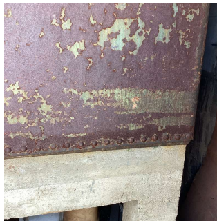
Roof 1 - Tank Room
