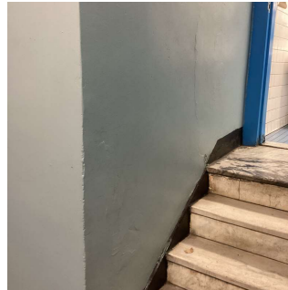
Corridor near Room 363
