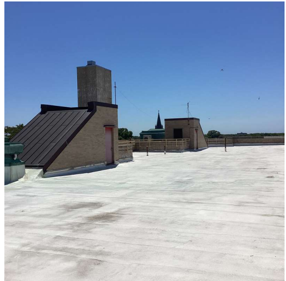
Roof 1 - Southwest view
