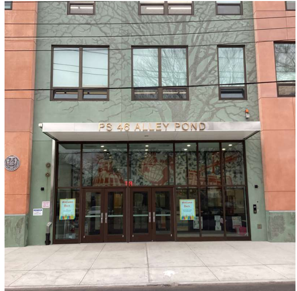
Facade A - 218th Street
