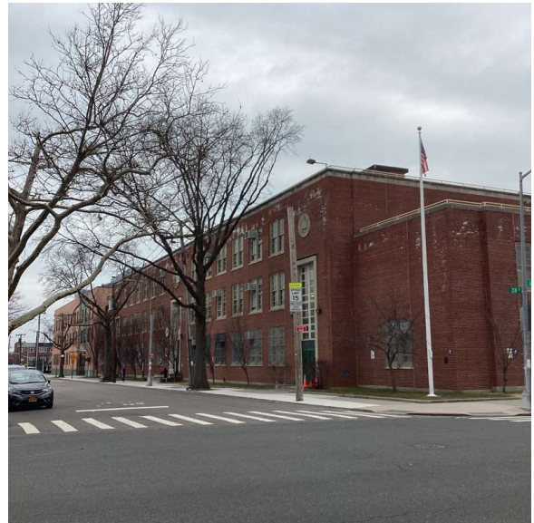
Corner of 218th Street and 67th Avenue - Northeast view
