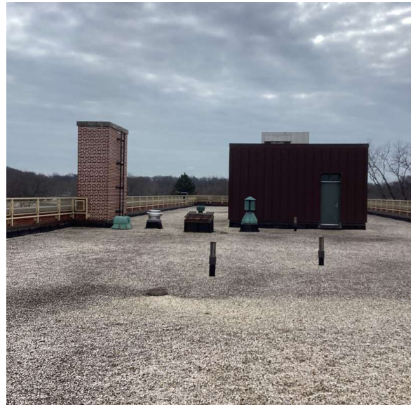
Roof 1 - Southeast view
