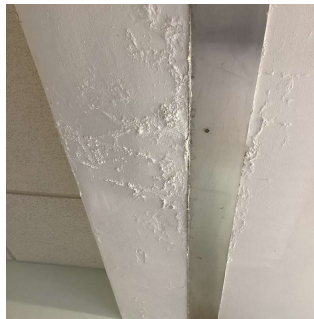
Roof 1 - Corridor near Stair C/3, also Roof 4 - Room 122 No violations recorded.
