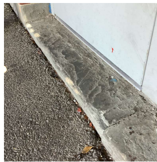
Facade B - Exit 3
