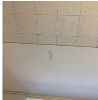
Corridor near Stair E/2
