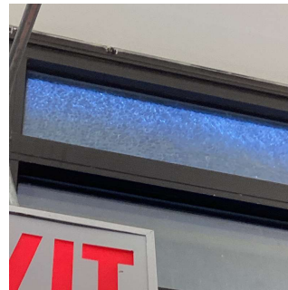
Facade C - Exit 4
