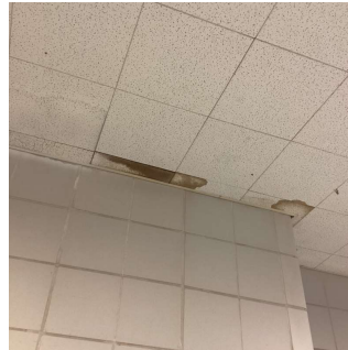
Corridor near Stair G/2
