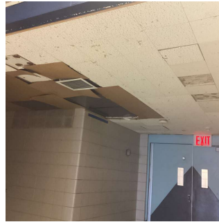
Corridor near Room 414
