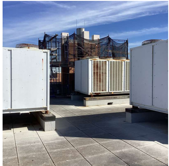
Roof 1 - Northeast view
