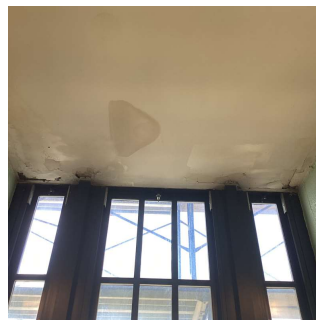
Corridor near Stair C/3
