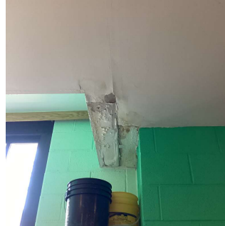
Roof 1 - Library (two locations)
