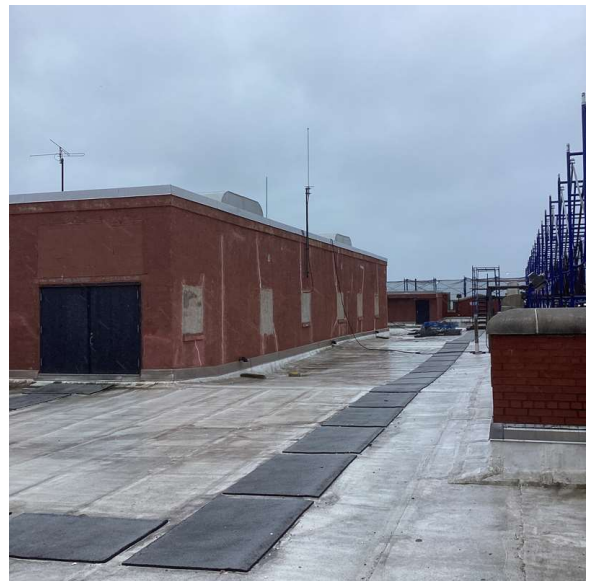
Roof 1 - Southeast view
