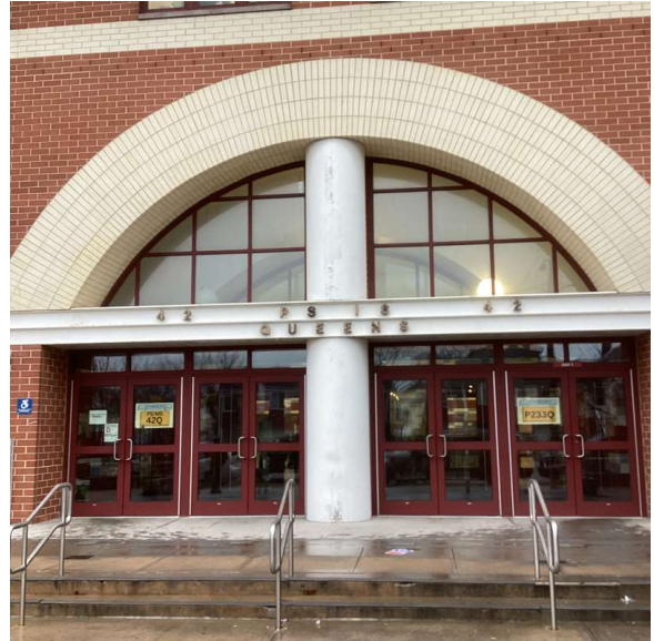
Facade B - Beach 66th Street
