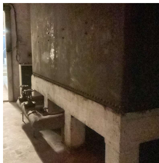
Roof 1 - Penthouse No violations recorded.
