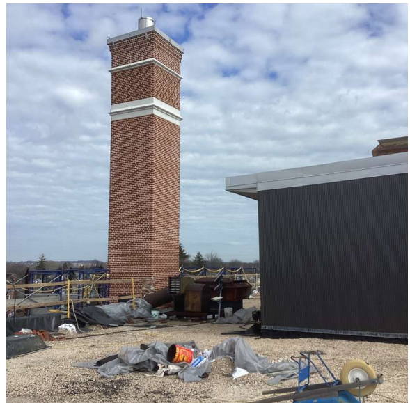
Roof 1 - Northeast view
