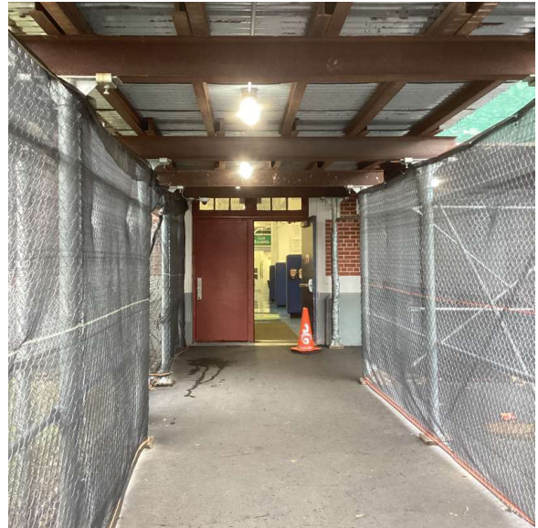
Facade A - Everitt Place
