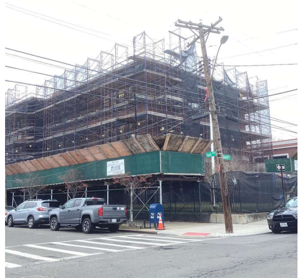
Corner of Foch Boulevard and Everitt Place - West view
